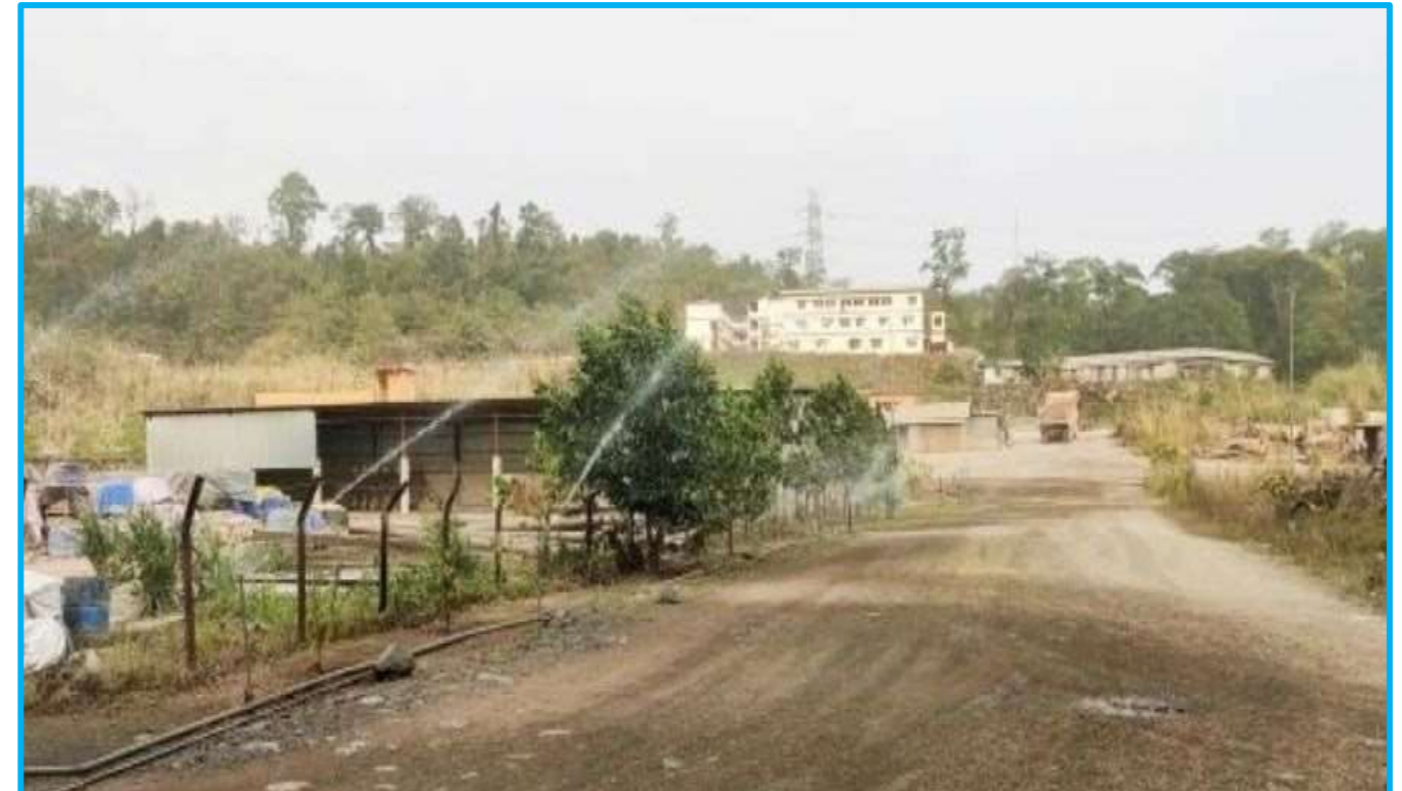
Water Sprinkling through Permanent Water Sprinklers at Transportation Roads
