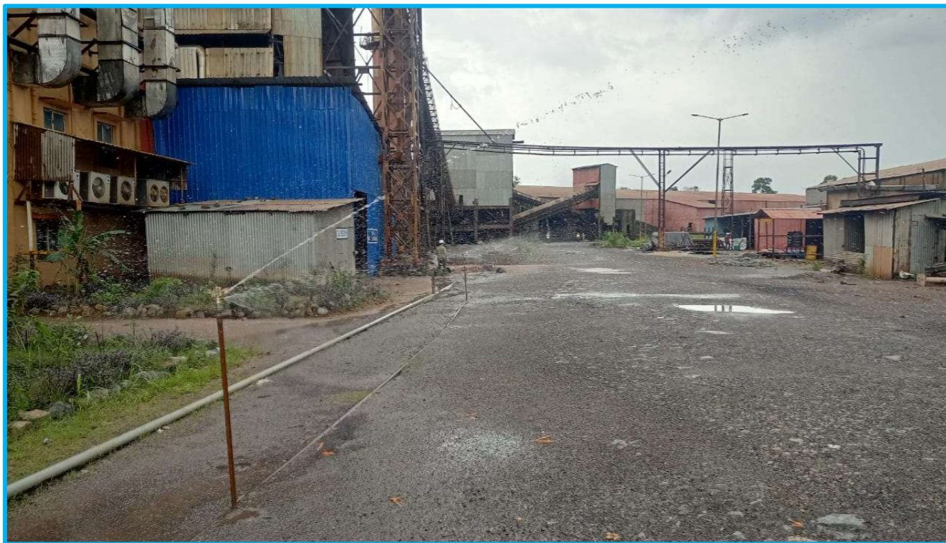
Water Sprinkling through Permanent Water Sprinklers at internal Road at CPP
