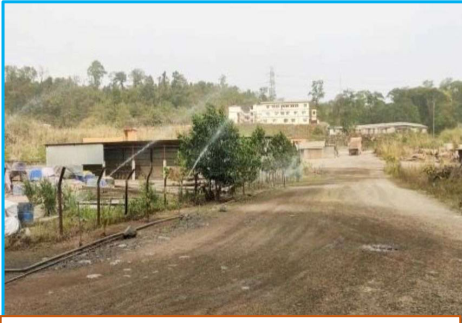
Water Sprinkling in roads through Permanent Water Sprinklers
