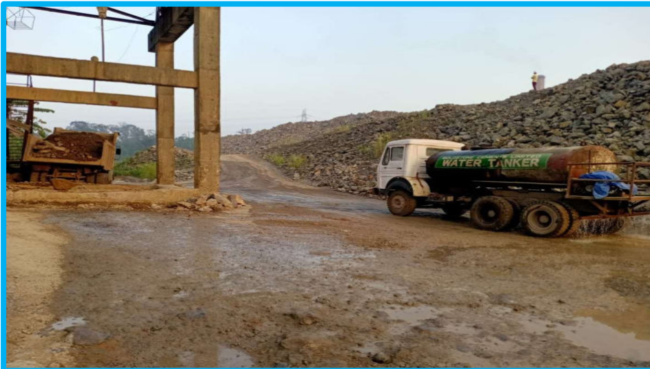
Water Sprinkling through Water Tanker In all internal Roads at Plant
