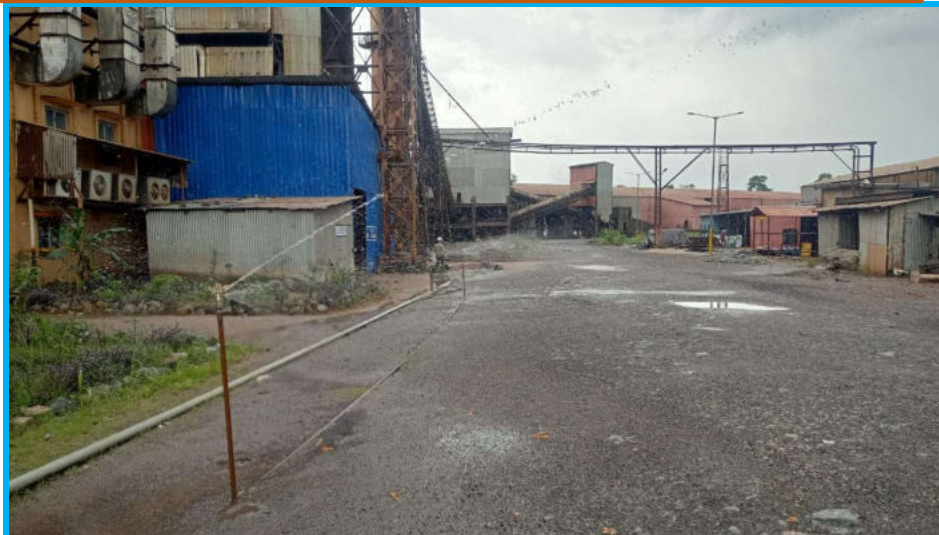
Water Sprinkling through Permanent Water Sprinklers
