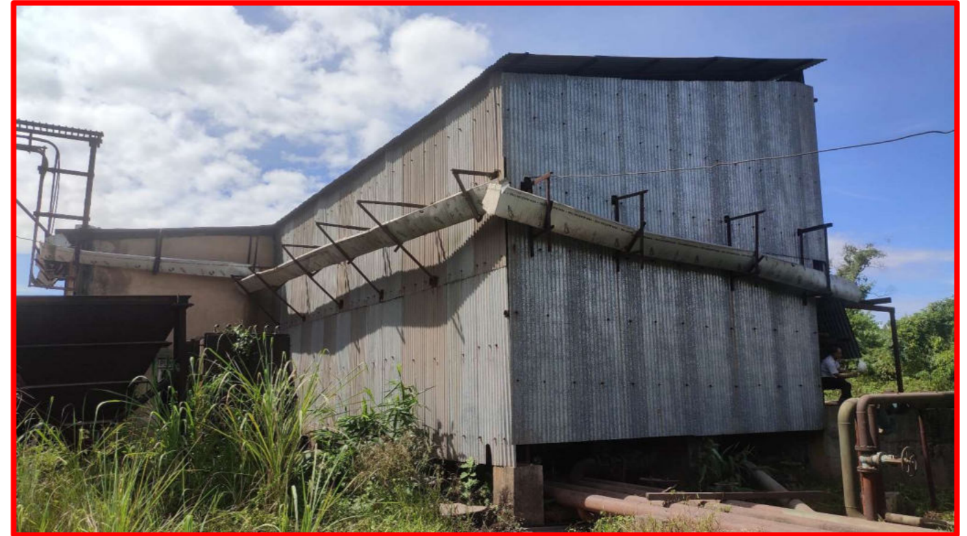
Rooftop rainwater collection and harvesting system at CPP water reservoir
