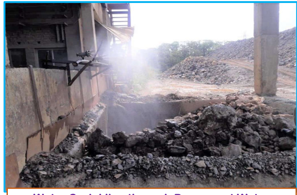
Water Sprinkling through Permanent Water Sprinklers at Limestone Crusher
