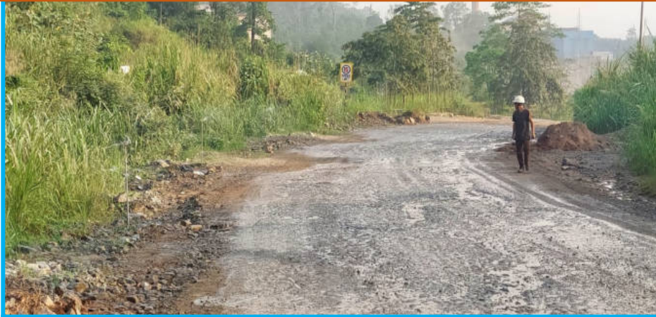
Water Sprinkling through Permanent Water Sprinklers from main Security Gate to HSD Pump
