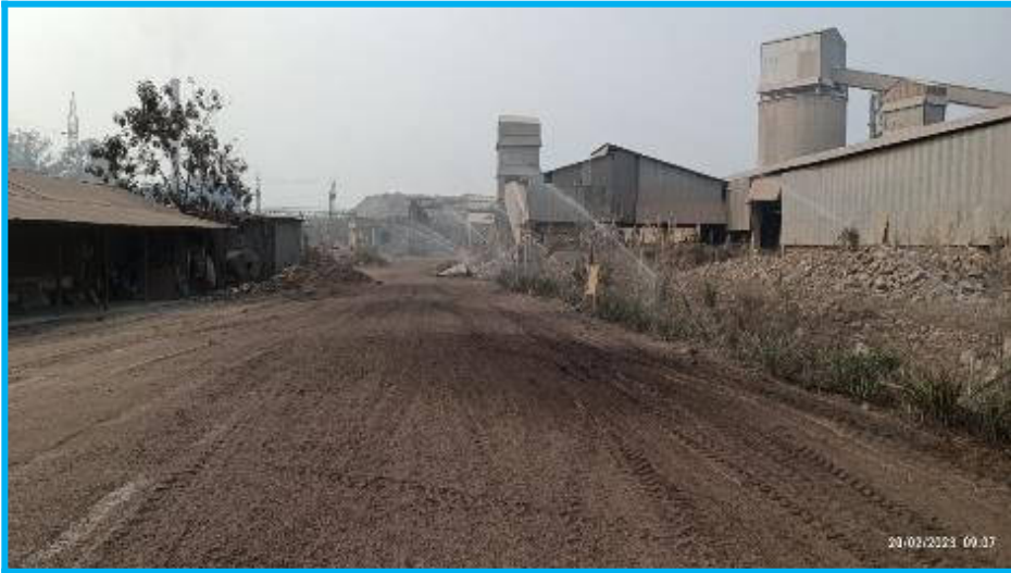
Water Sprinkling through Permanent Water Sprinklers from CIVIL office to MRSS
