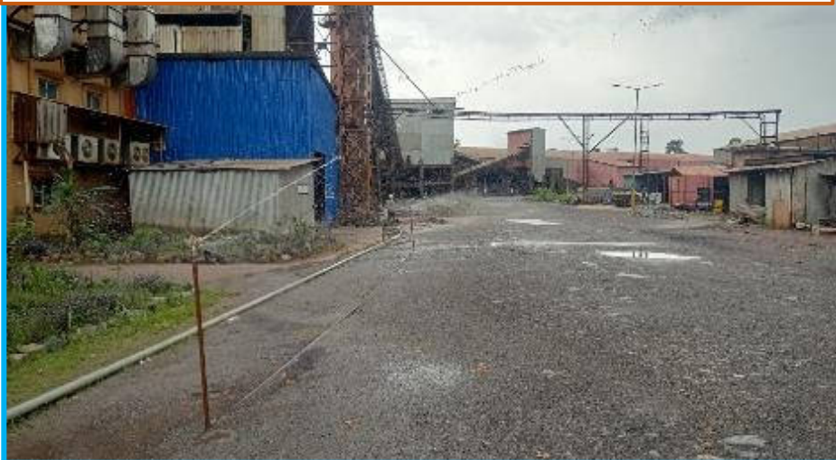
Water Sprinkling through Permanent Water Sprinklers at CPP road
