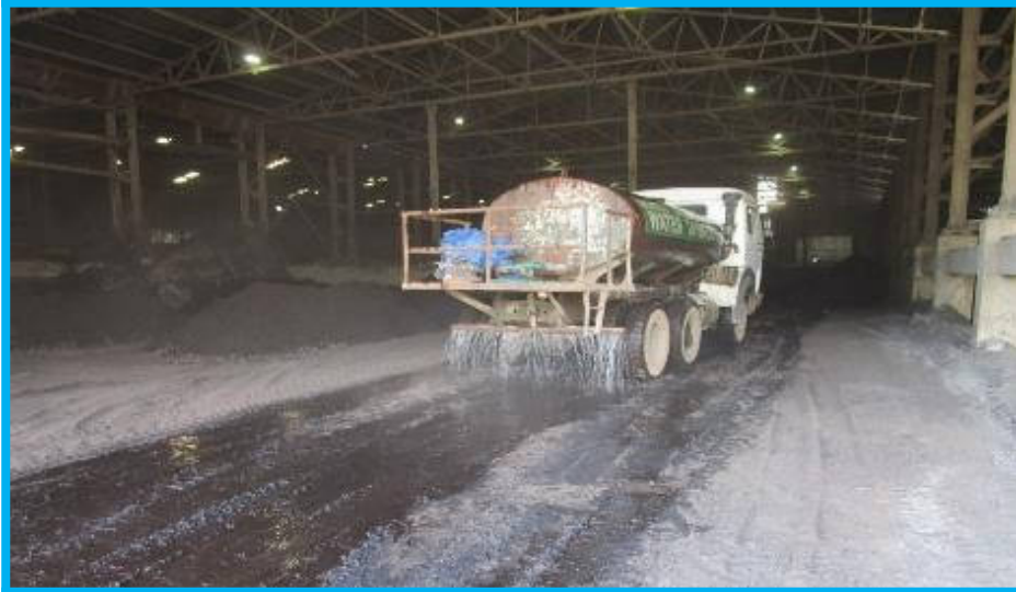
Water Sprinkling through Water Tanker Inside the coal storage sheds
