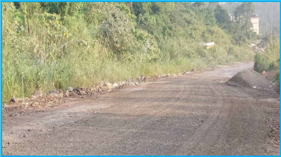
Water Sprinkling through Permanent Water Sprinklers from main Security Gate to HSD Pump
