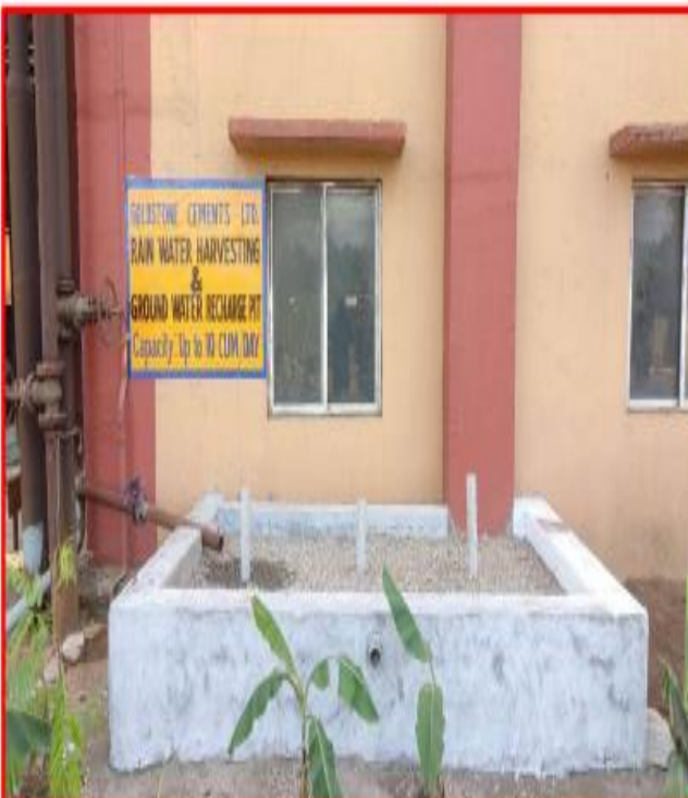
Rooftop rainwater collection and ground recharge system at CPP
