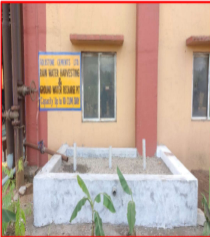
Rooftop rainwater collection and ground recharge system at CPP
