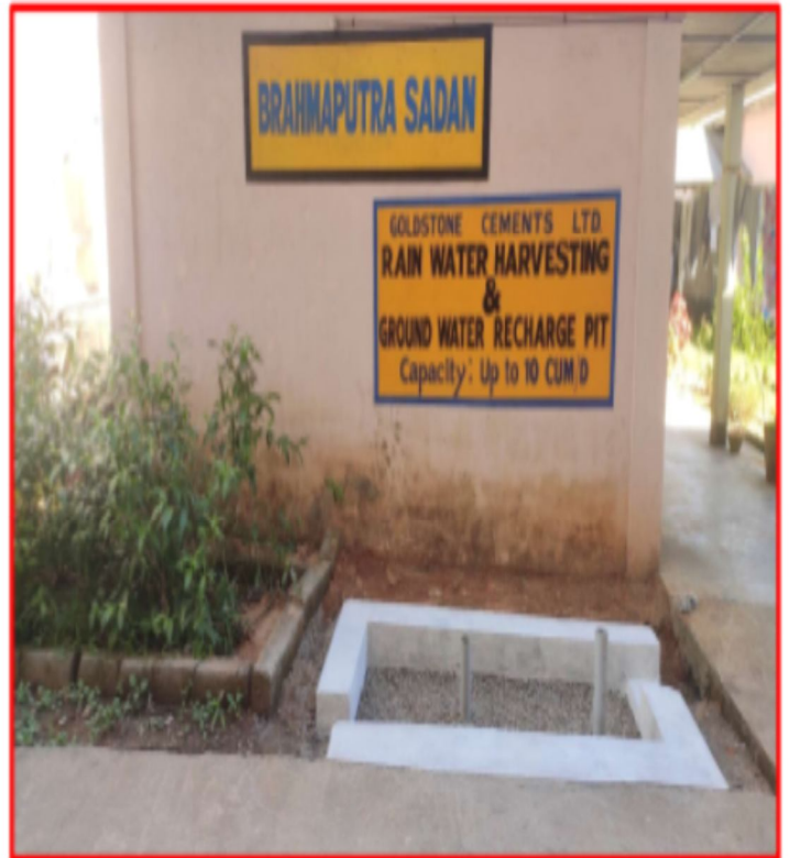
Rainwater collection and ground recharge system at Guest House (Brahmaputra Sadan)
